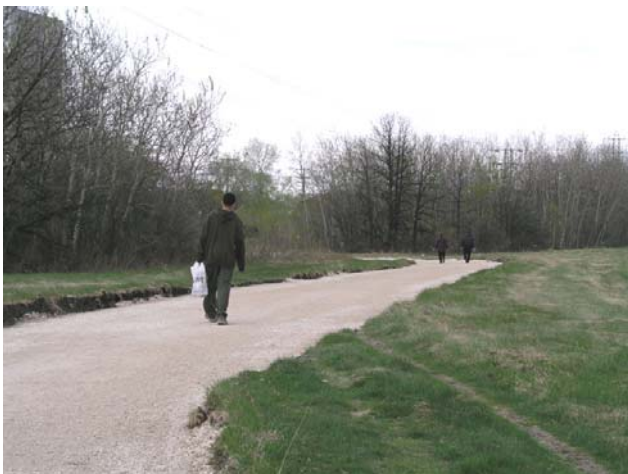
Crushed gravel surfacing awaiting asphalt in summer of 2006
